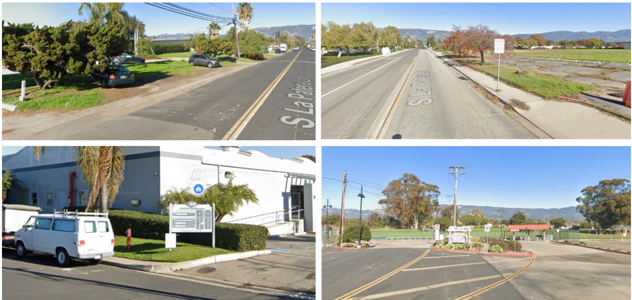
Figure 2-33. S La Patera Lane Sidewalk Conditions: (a) Missing Sidewalks, (b) Limited Shade, (c) Missing Curb Ramp, (d) No Signage.
