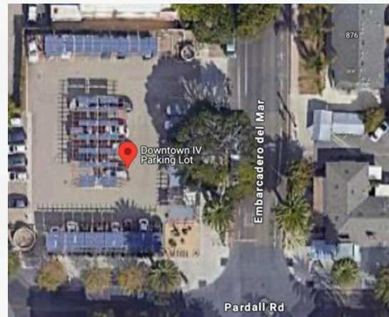
Solar Parking Lot
