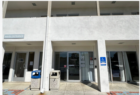
Community Room exterior
